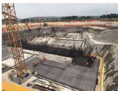
JULY 7, 2025 WORKS ON THE QUILONGA WATER SUPPLY SYSTEM PROGRESS
